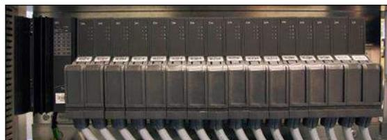
There are two series of the ACN I/O units: M80 and M120. M80 series includes units for a low current/voltage analog/digital applications. M120 series units are used when high voltage isolation between the channels is needed or when digital interface is needed for high DC/AC line voltages without external relays.
